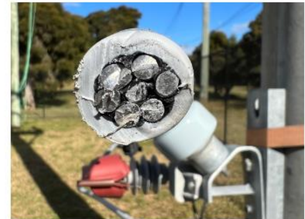
Covered conductor is designed to reduce unplanned outages and the likelihood of powerlines starting bushfires.
